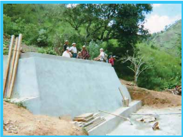
The water project nearing completion.
