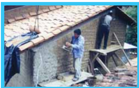
Building the chapel at Chipuerta.
